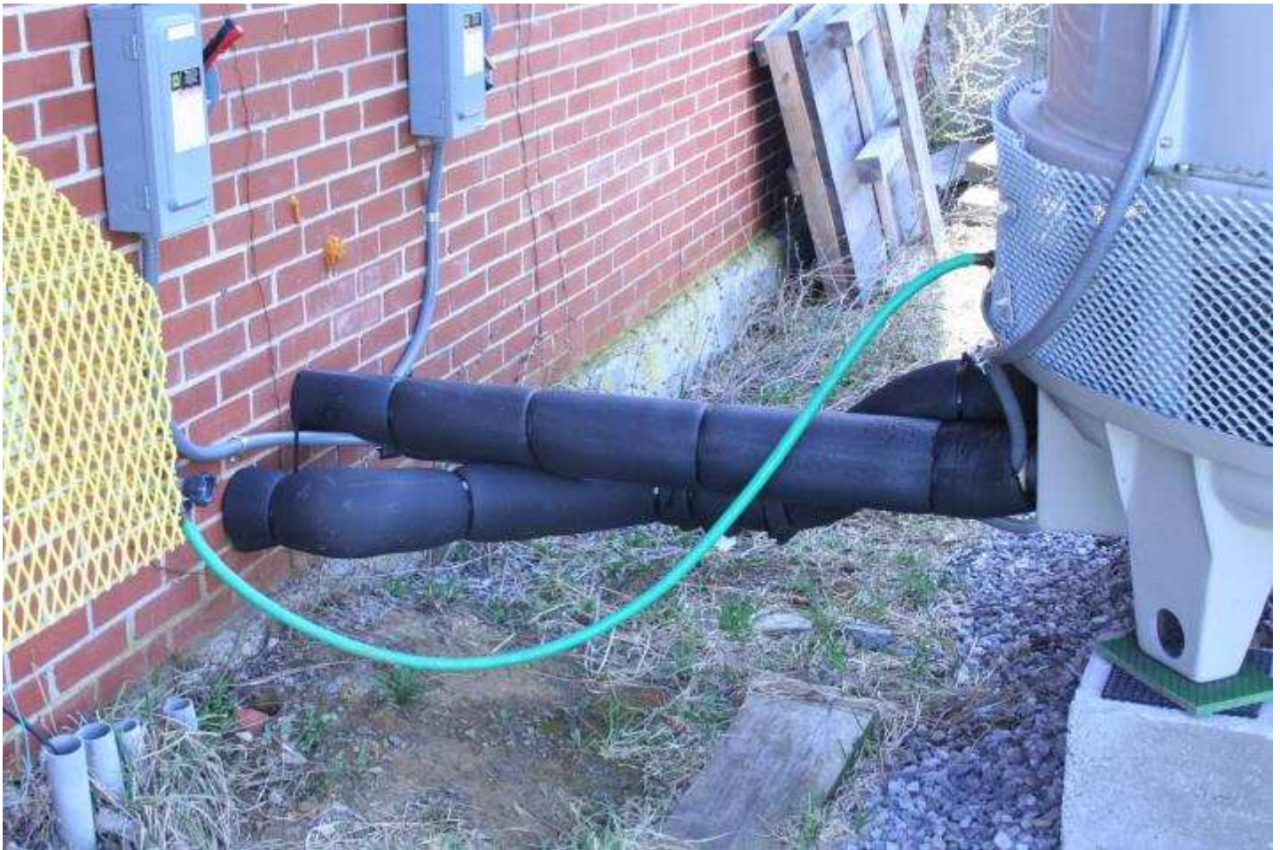
Figure 33. Picture of the added insulation on the cooling tower pipes
