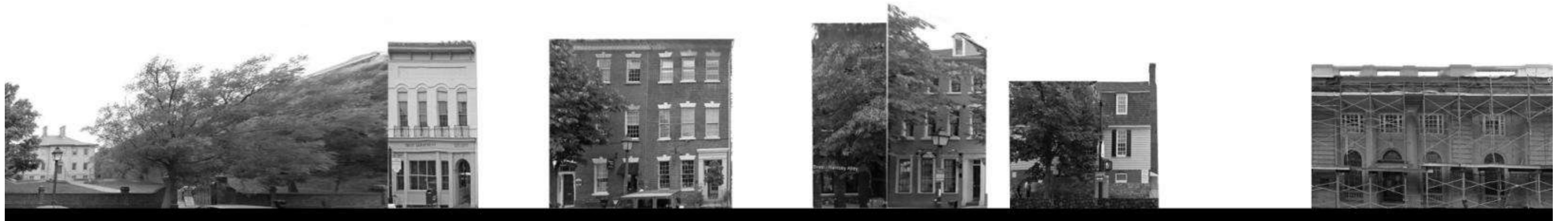
Existing West Elevation from Fairfax Street
