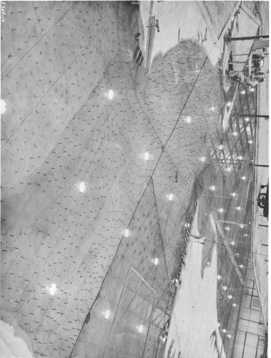
Fig. 4. James River hydraulic model showing Hampton Roads (looking seaward) with Newport News on the left and Norfolk on right. (Note Craney Island Disposal Area intruding on right and tidal programmer upper left.) (Courtesy of U.S. Waterways Experiment Station, Vicksburg, Mississippi.)
