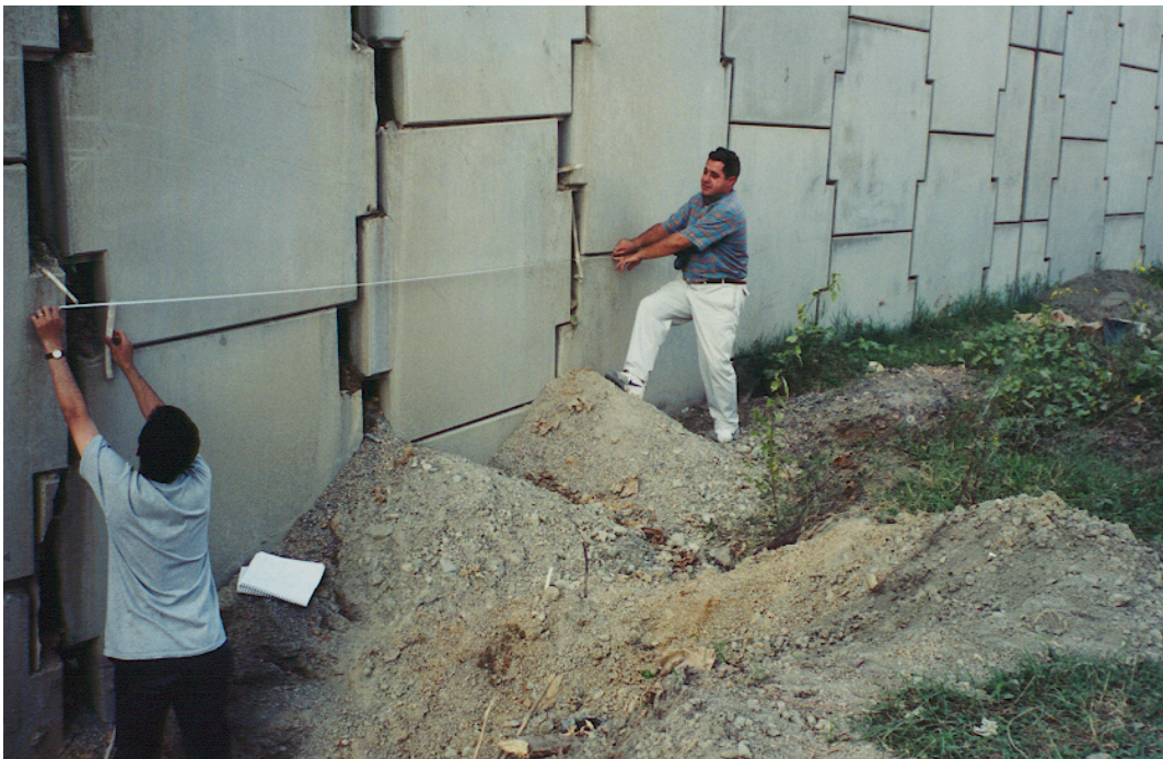
Figure 2-11. Separation of the facing panels due to vertical distortion and spilled backfill material
