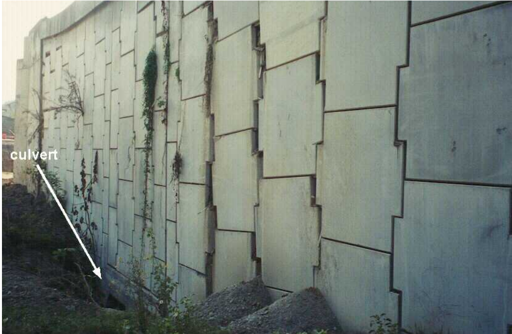
Figure 2-10. Distorted facing panels near the culvert
