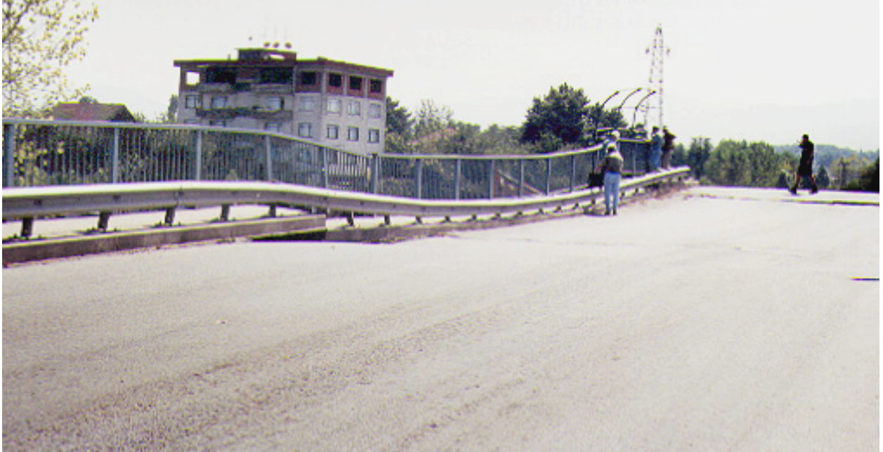
Figure 2-14. Damage at the top of the approach embankment. Sagging due to foundation settlement and cracks in the pavement are evident.
