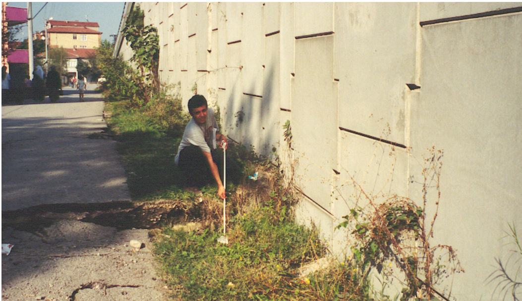
Figure 2-9. Settlements and ground cracks near the buried culvert
