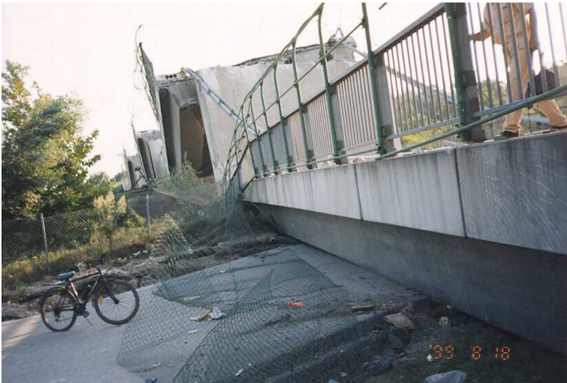
Figure 2-7. Collapsed bridge decks
