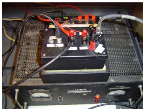
Figure 4-10. Circuit box and power supplies used to power the electromagnet
