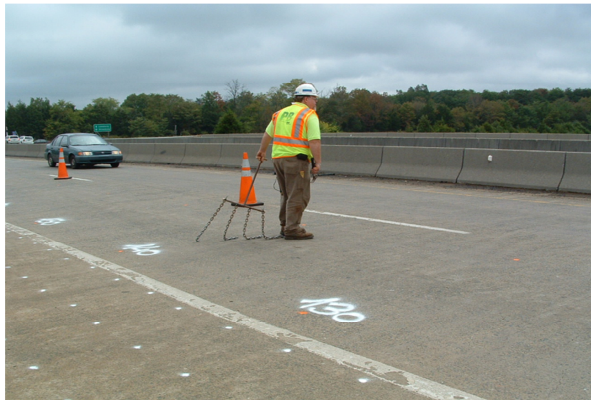
Figure 29 – Deck Chain Dragging
