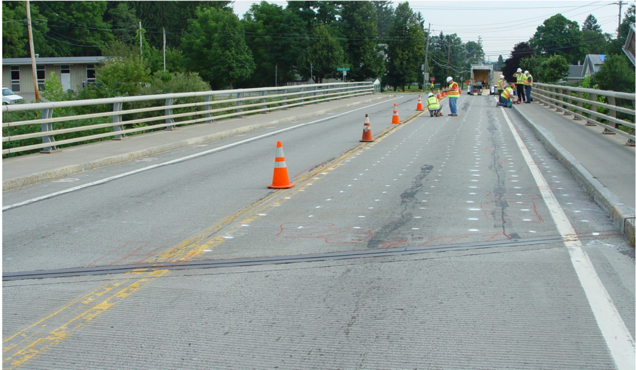
Figure 113 – View of Deck Surface
