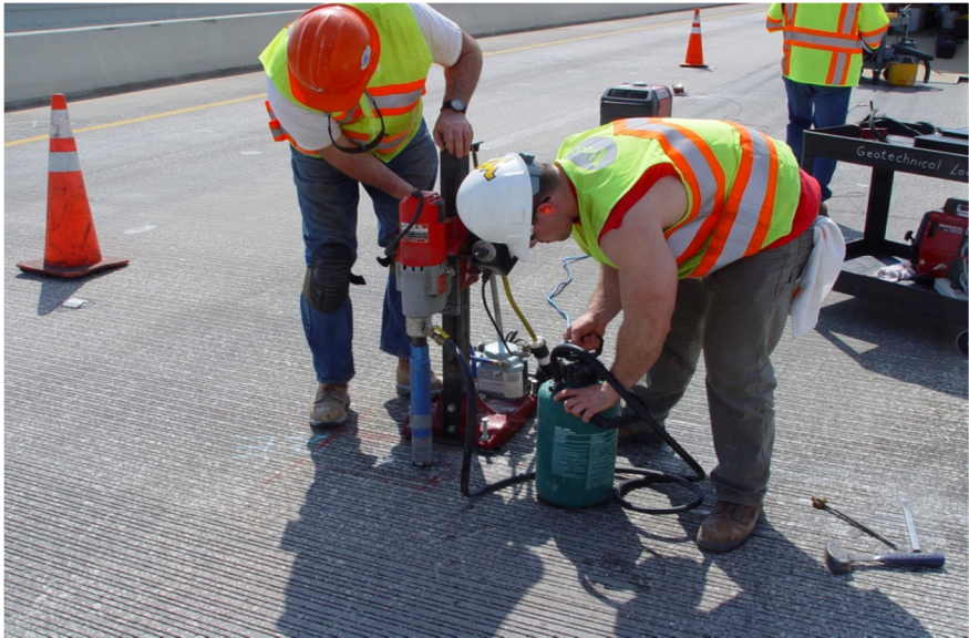
Figure 66 – Concrete Coring using Handheld Equipment
