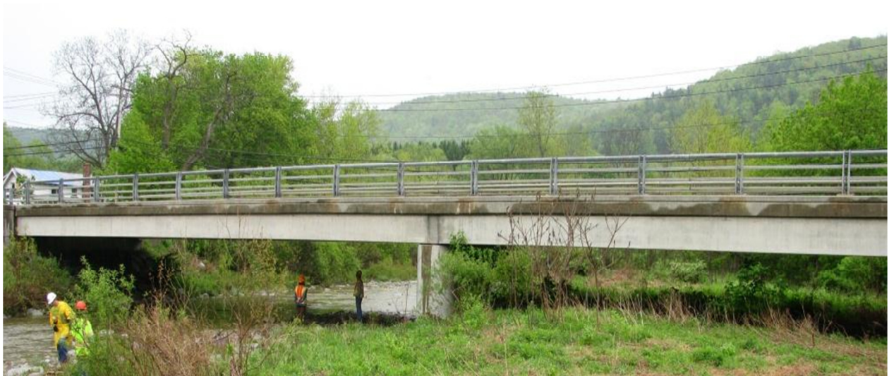
Figure 112 – Route 21 Bridge over Karr Valley Creek
