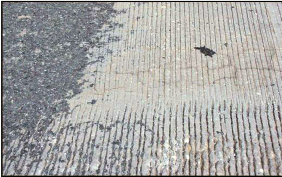
Figure 60 – Visual Inspection – Map Cracking
