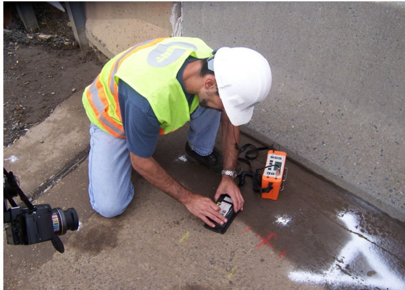
Figure 30 – Cover Depth Measurements Being Taken
