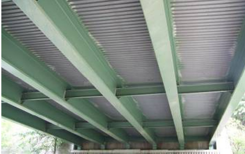
Figure 83 - View of Steel Girders and Stay-in-Place Forms
