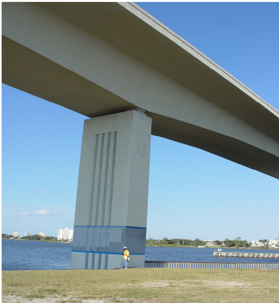
Figure 59 – Side View of Pier and Prestressed Box Beam
