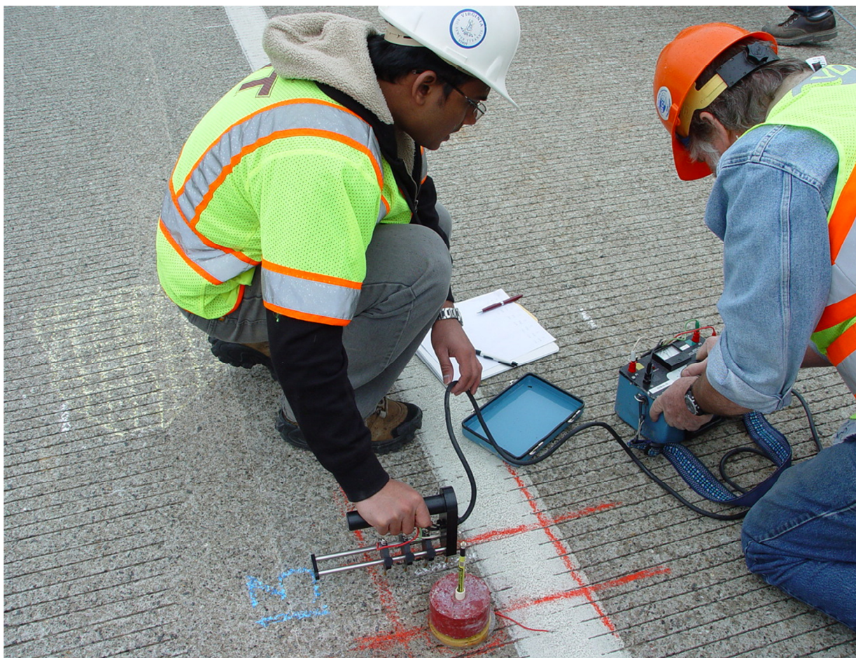
Figure 89 – Measurement using Four-Point resistivity Meter
