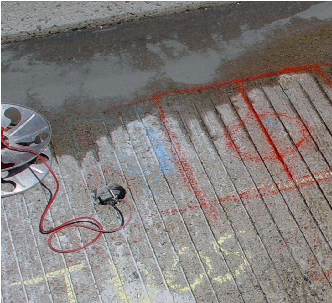
Figure 86 – Continuity Test on Bridge Deck
