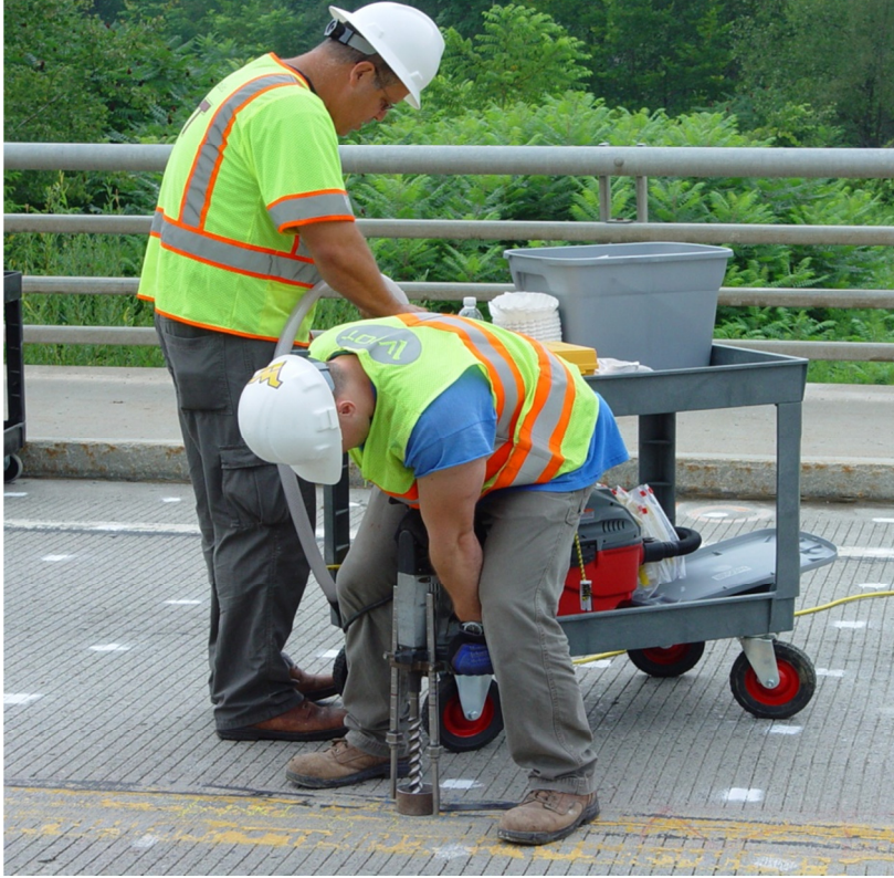
Figure 117 – Chloride Sampling Process
