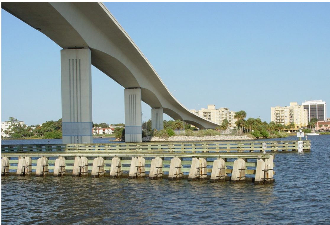
Figure 58 – Seabreeze Bridge over Halifax River
