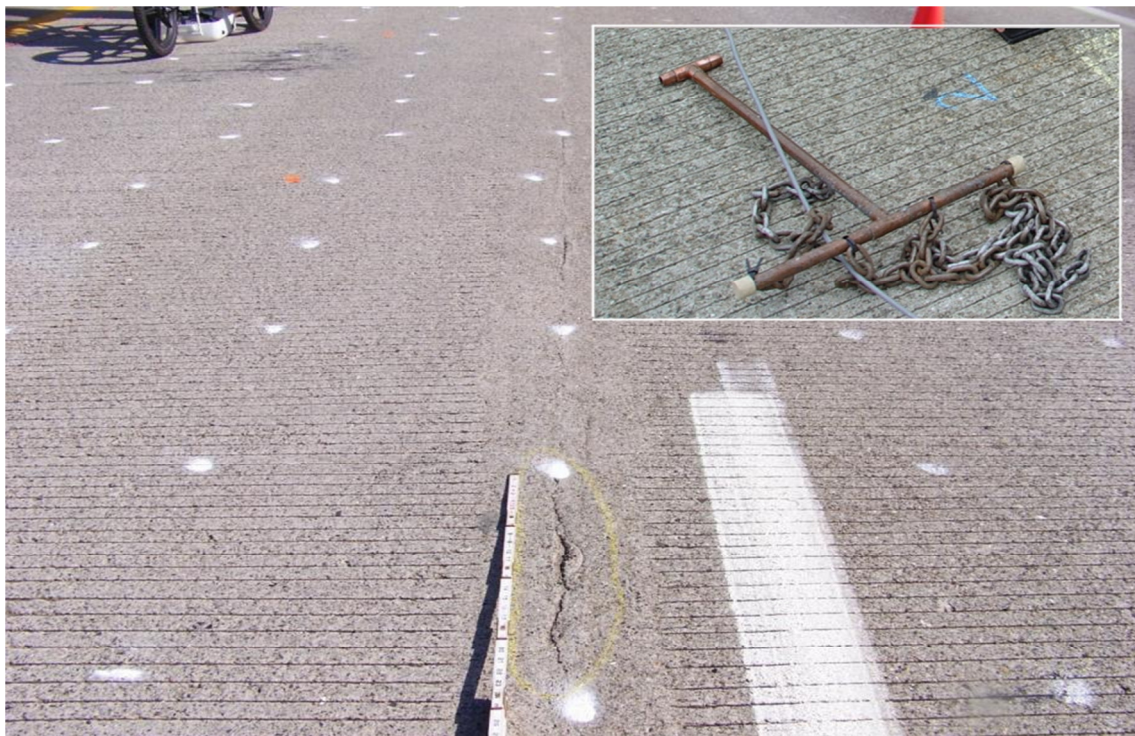
Figure 84 – Visual Survey of Cracks and Chain Dragging Equipment
