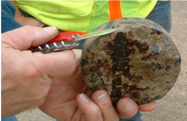
Figure 38 - Core Showing Cracking Over Corroded ECR
