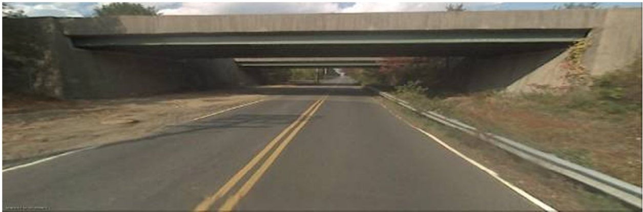
Figure 82 – I-165 Bridge over Sharon Station Road
