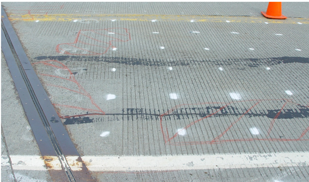
Figure 114 – Marking of Delamination Locations Using Sounding Techniques
