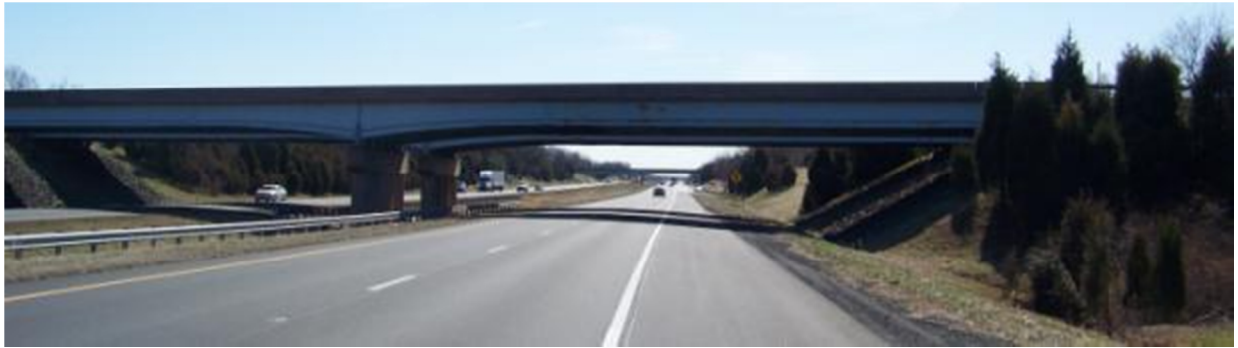
Figure 27 – U.S.-15 Bridge over I-66
