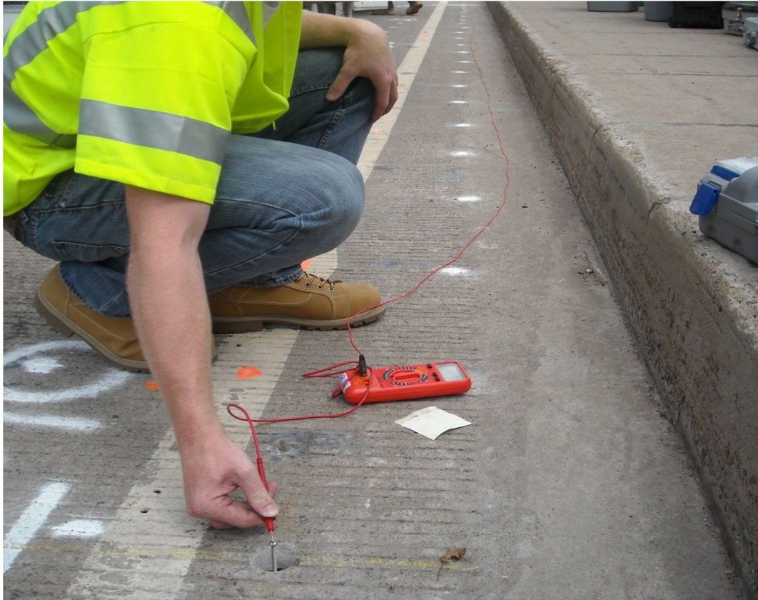
Figure 33 – Continuity Test on Bridge Deck
