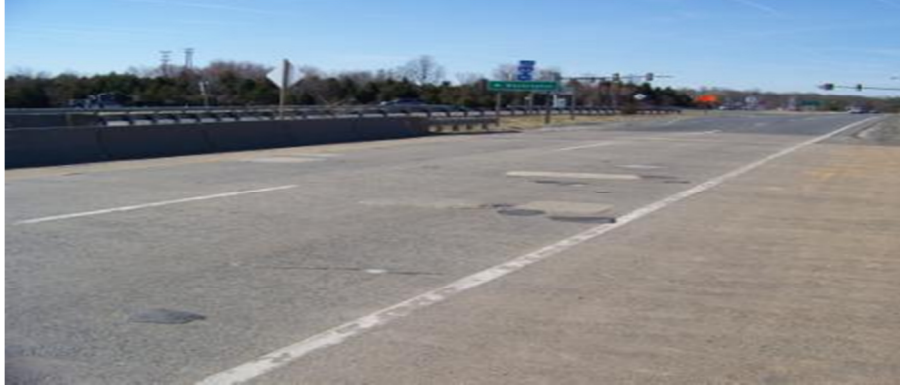
Figure 28 – U.S. Route 15 Southbound Deck
