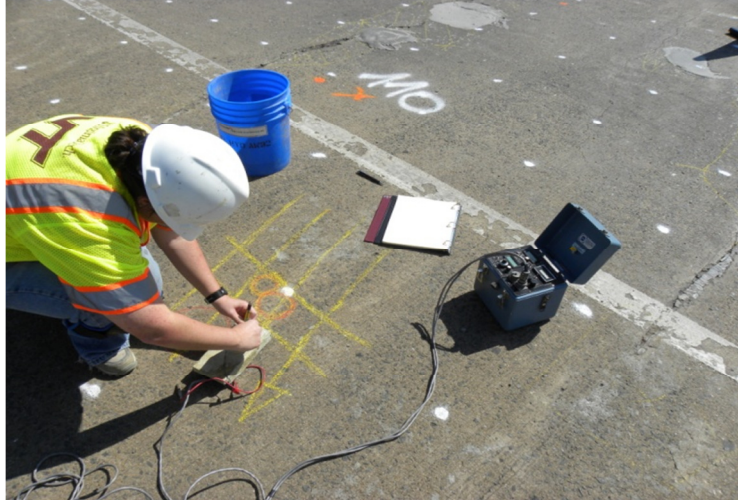
Figure 35 – Corrosion Rate Testing with 3LP Device
