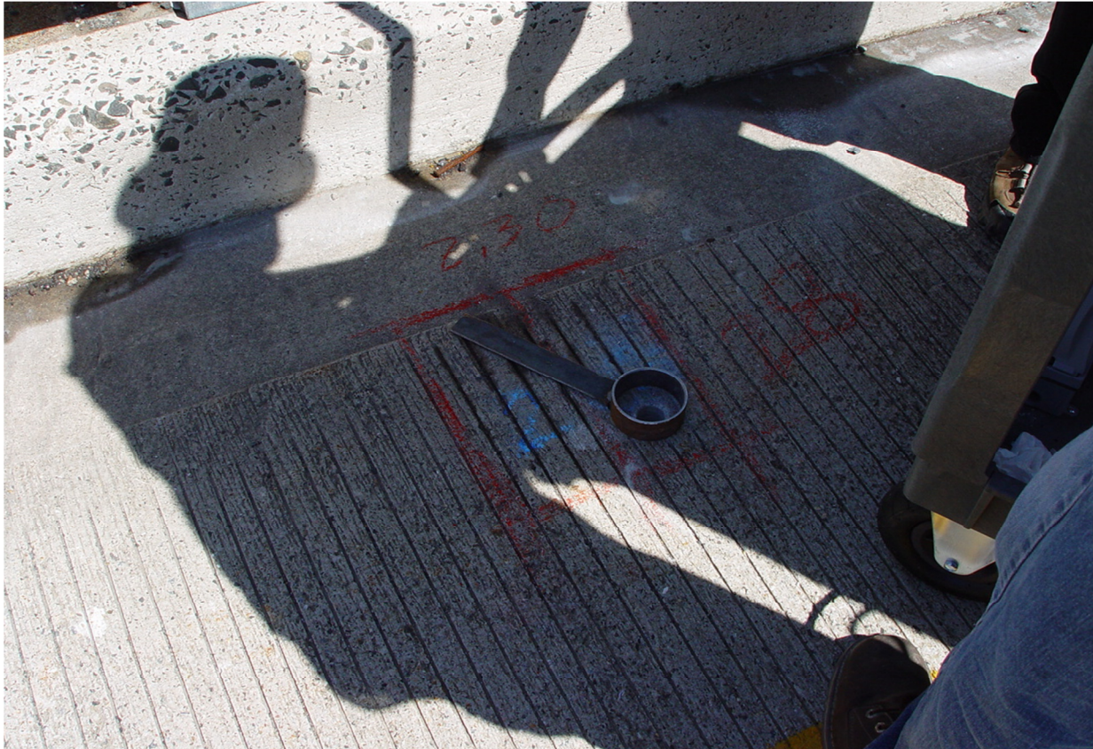
Figure 90 – Drilling to Collect Chloride Samples
