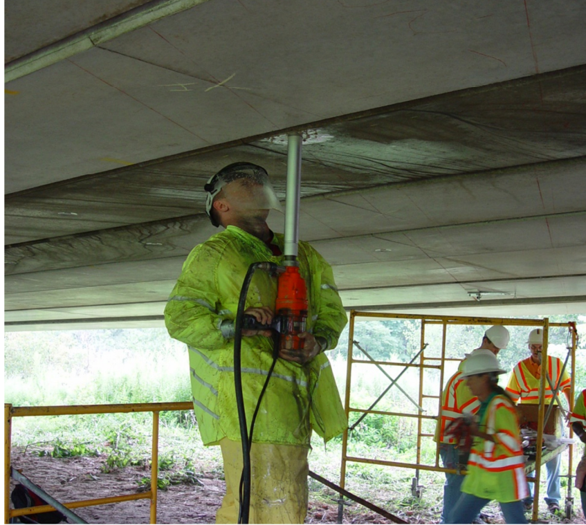
Figure 118 – Concrete Coring at Bottom of Bridge Deck
