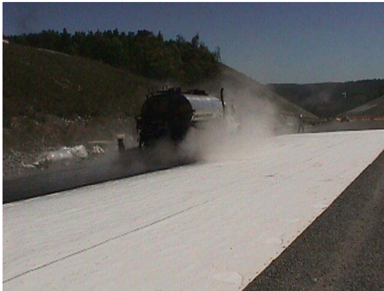
Figure 2-2. Prime Coat Application on Top of the Geocomposite Membrane in Section J
