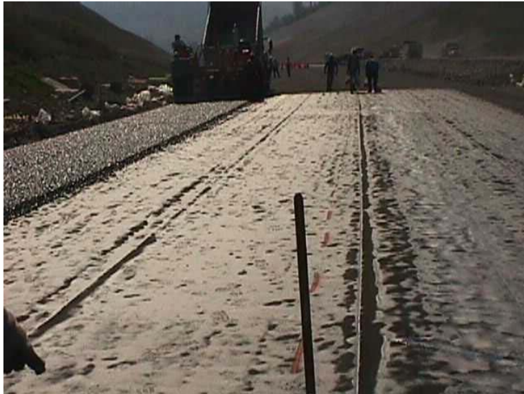
Figure 2-3. Installation of the Open-Graded Drainage Layer in Section J
