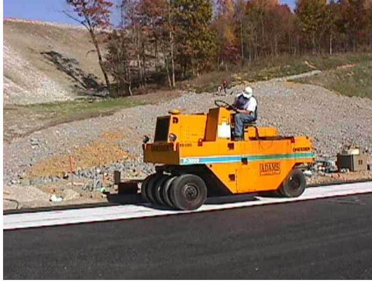
Figure 3-4. Compaction of the Geocomposite Membrane in Section K
