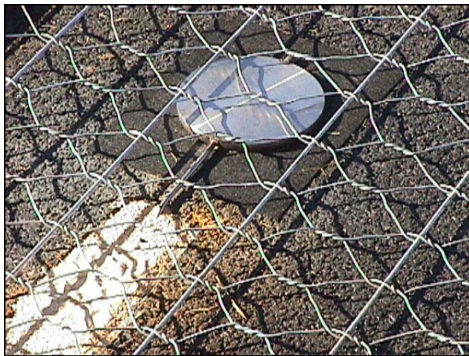
Figure 4-3. Pressure Cell Installation Covered by Steel Mesh
