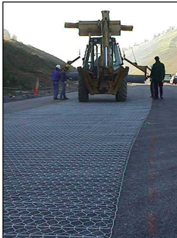
Figure 4-5. Passage of a Roller on Top of the Steel Mesh to Relieve the Natural Curvature of the Roll
