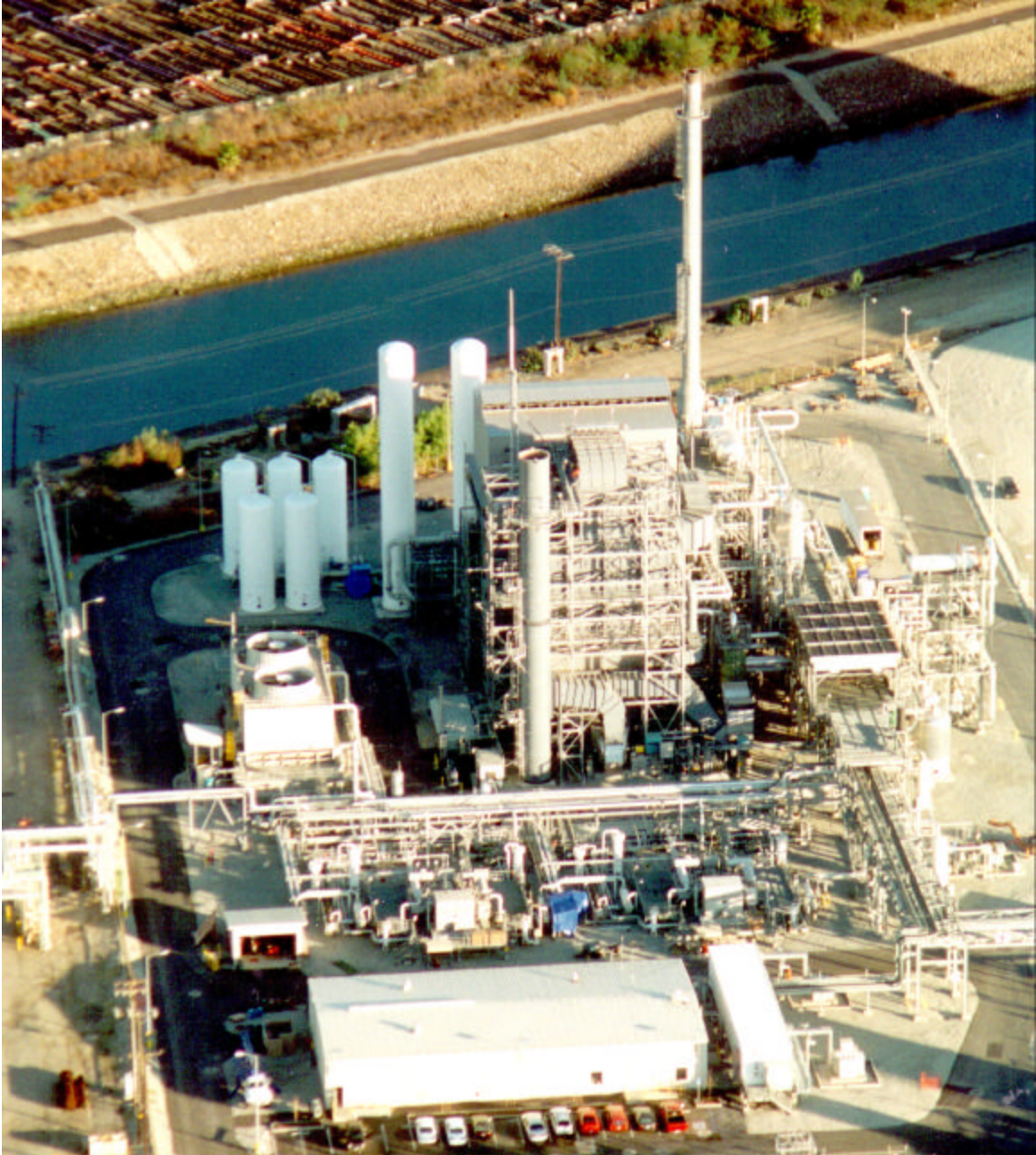
Figure 1.2: Air Product's Carson, CA hydrogen plant, 237 tonnes per day of hydrogen
