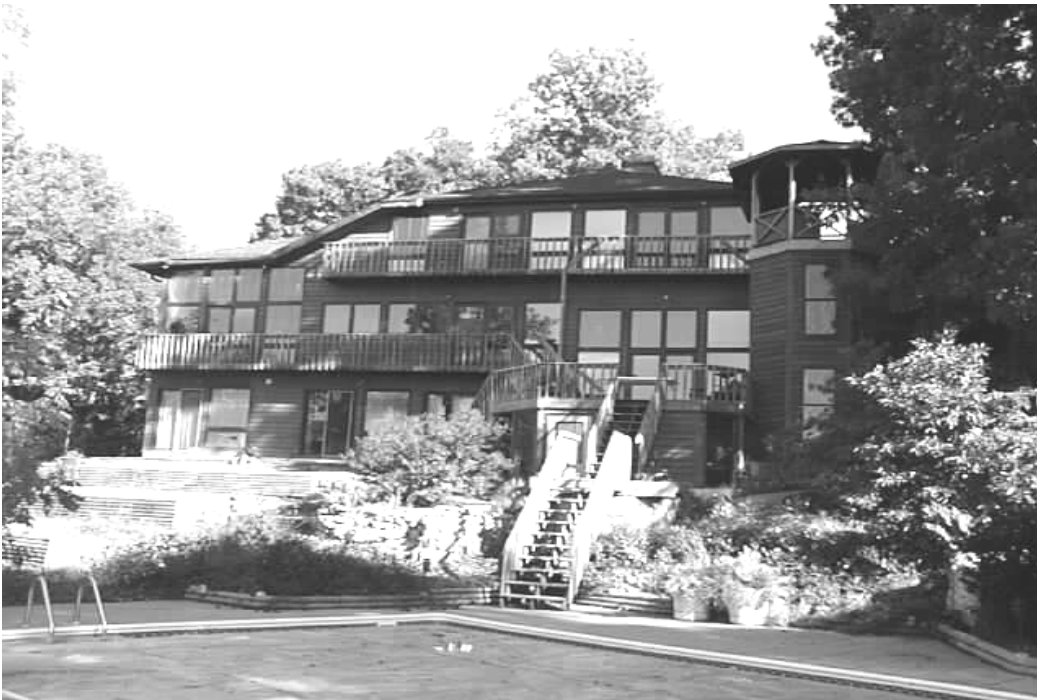
Figure 4- 1: The Beliveau house south elevation
