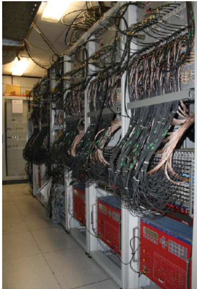
Figure 3.30: A few of the fourteen inner detector electronics racks. From top to bottom: PMT cables entering from the SSS, patch panel, FE power supply, adder/scaler module, FE crate and boards, Laben crate and boards, HV crate. See text for functional description.
