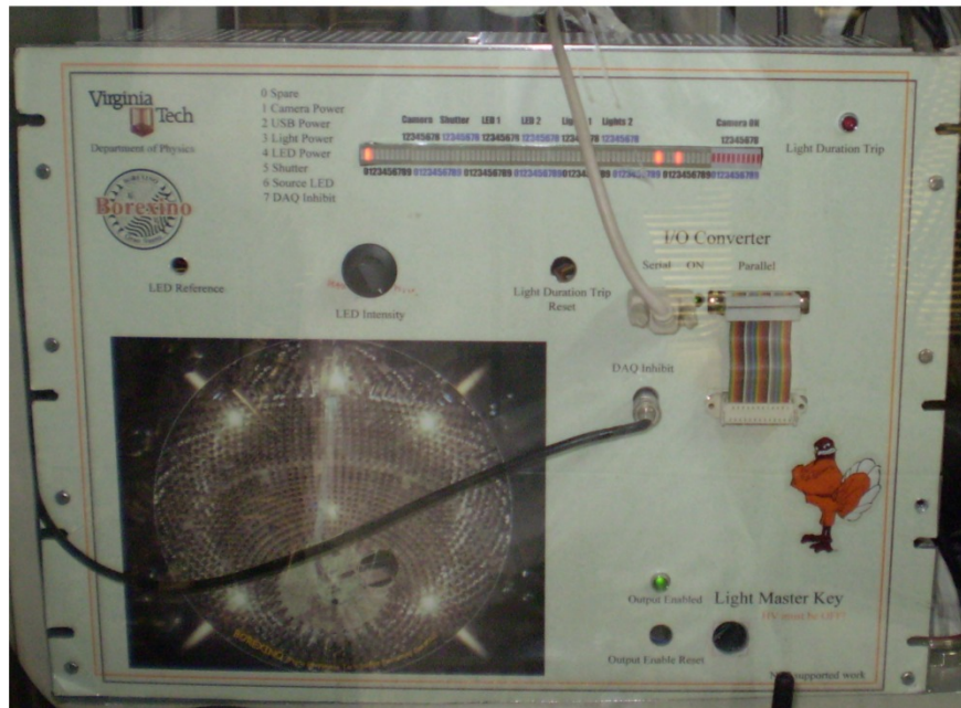
Figure 5.6: The camera system interface box in the computer cabinet in CR4. The box houses power supplies, relays, and interlocks for controlling the lights, LEDs, power, and picture taking ability for all of the cameras. A series of status LEDs along the top of the box are used to give visual feedback of which lines are drawing current. The original design of the system used an LED inserted with the source, the intensity of this LED would be controlled by the potentiometer knob on the front of the box, in its current implementation this is unused. The interlock for the quartz bulbs and the output enable switch have been moved to an enclosure accessible by shifters in the cleanroom.
