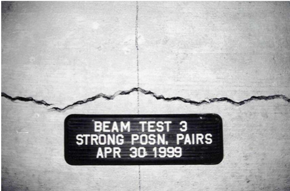
Fig. 7.14 Beam Test 3 with Large Crack Transverse to the Beam
