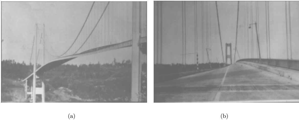
Figure 1.1: The Tacoma Narrows bridge before failure exhibiting large twisting motions. (a) Side view and (b) end view. Obtained from the internet site: http://www.fen.bris.ac.uk/engmaths/research/nonlinear/tacoma/tacoma.html .
