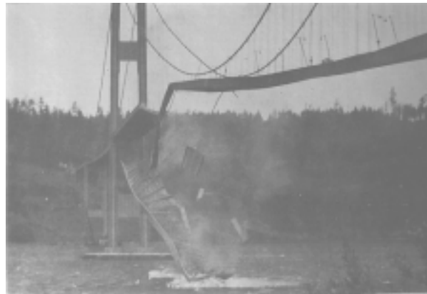
Figure 1.2: A side view of the Tacoma Narrows bridge tearing apart. Obtained from the internet site: http://www.civeng.carleton.ca/Exhibits/Tacoma_Narrows/DSmith/photos.html .
