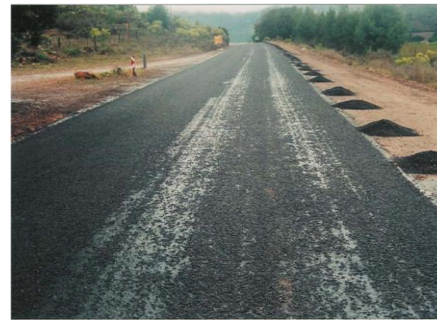
Figure 9-4 Early failures due to lack of adhesion and climate effects
