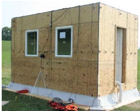
Figure 3.19: Photograph of the single-room structure.
