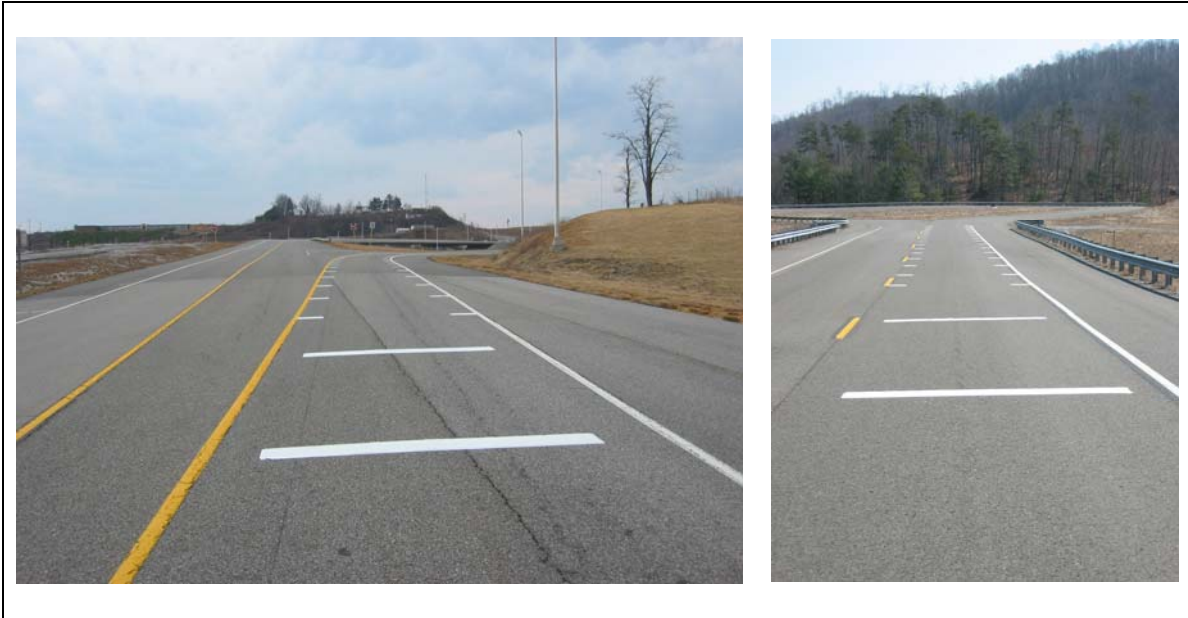
Figure 6-1: Peripheral transverse bars applied to the Smart Road at the ramp (left) and at the small loop (right)
