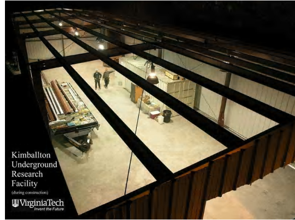
Figure 60 Kimballton Underground Research Facility (KURF) near Virginia Tech. S. Derek Rountree and R. Bruce Vogelaar in KURF during construction. The inclosure is 40'x100' and 20' high at the roof's peak.
