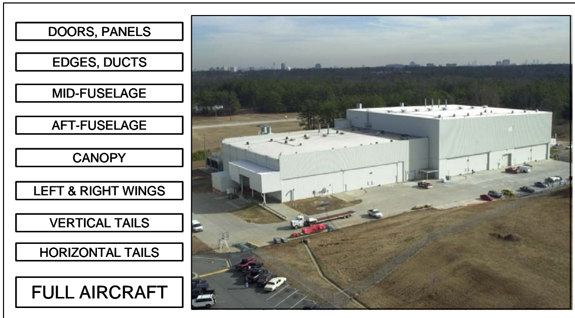
Figure 30. Major components and primary finishes facility, L-64.
