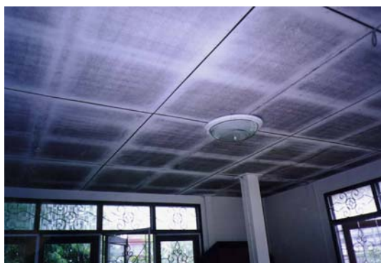
Figure 22. Molds in Bedroom
