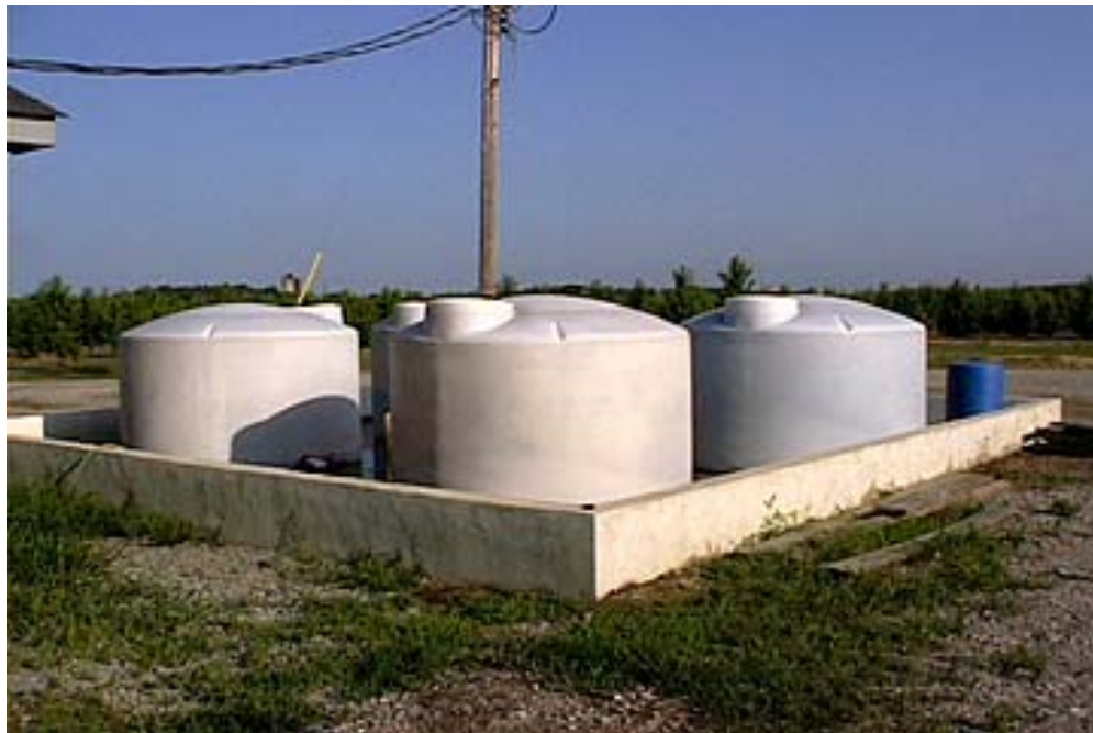
Figure II.6. Tanks store fertilizer for daily applications through the irrigation system.
