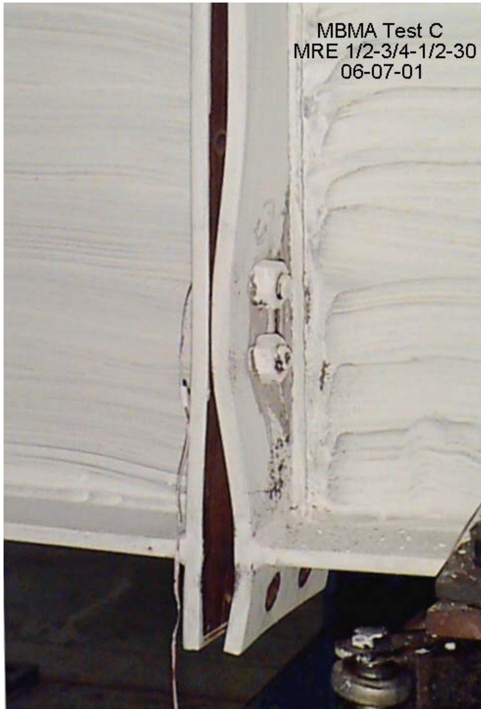
FIGURE 3.23: PHOTOGRAPH OF THIN PLATE FAILURE (TEST C-MRE 1/2-3/4-1/2-30)
