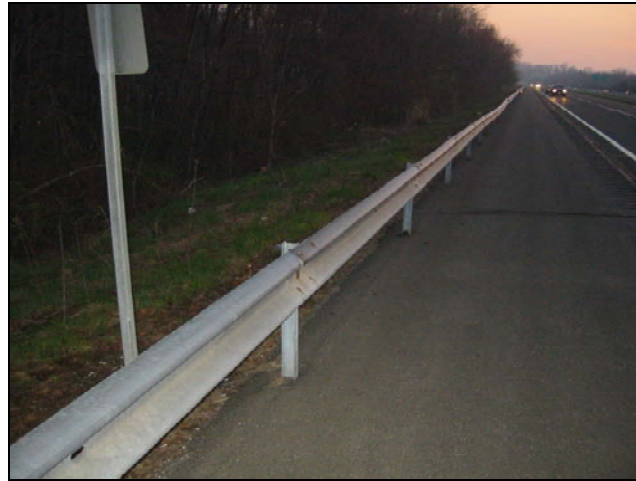
Figure 2. Roadside Hardware: Weak-Post W-Beam Barrier along I-87 in New York State [Douglas Gabauer, 7/7/2003]
