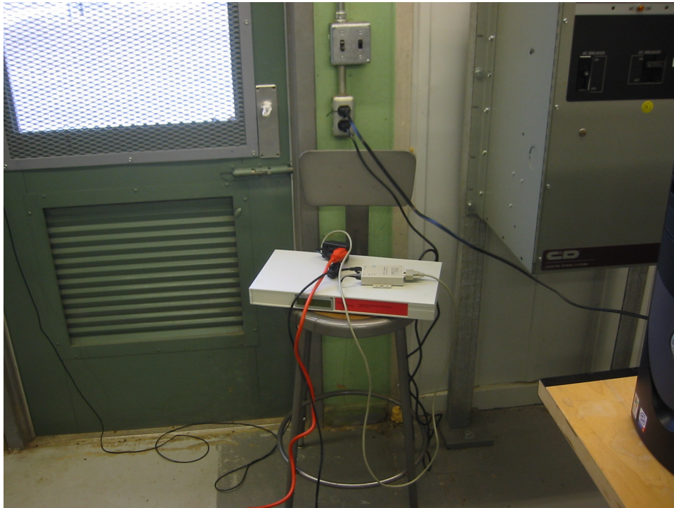
Fig 6-19. FDR plugs into 110 V outlet in Matt Funk 345kV substation's control room
