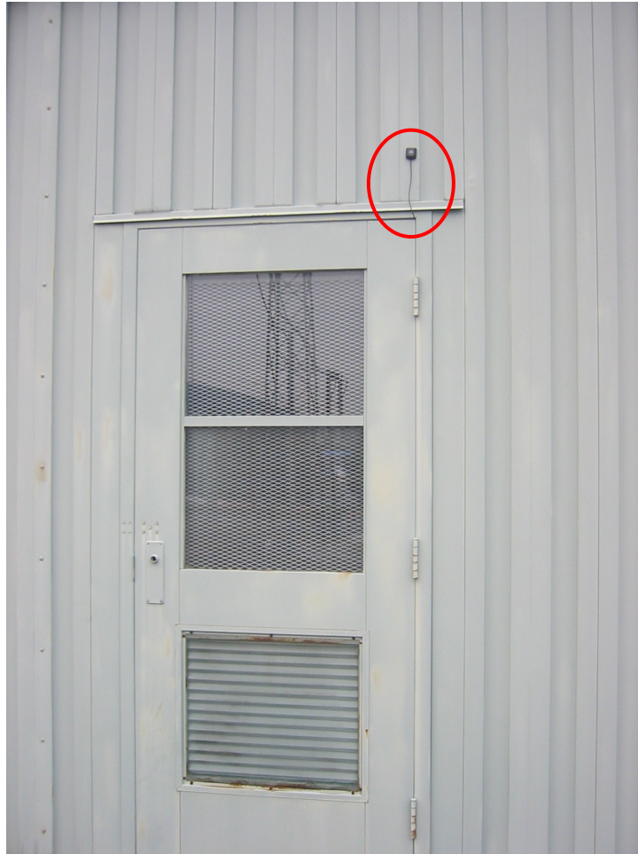
Fig 6-21. GPS antenna placement, circled in red.
