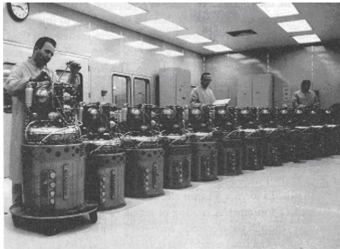
Figure 2-2. The AFCs fabricated for APOLLO space program (courtesy of UTC Fuel Cells). 2
