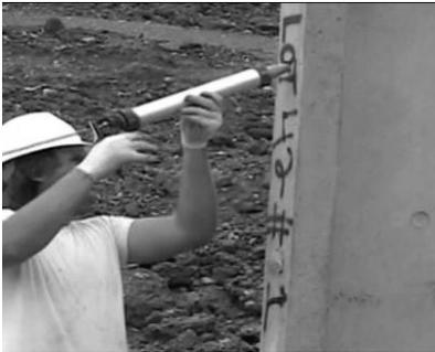
Apply polyurethane caulk on the upper surface of top ledgers and lift the first floor decks into place piece by piece
