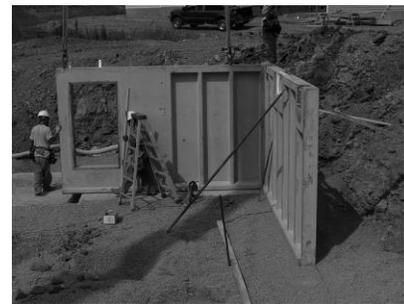
Bolt the walls together by three 12.7x140mm galvanized standard grade bolts per connection
