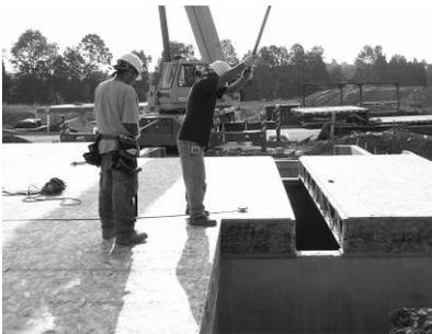
Bolt the sill plate of floor decks and the top ledger of the wall panels with 15.9mm lag bolts placed 305mm on center
