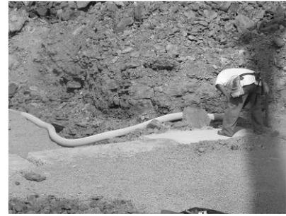
Tamp and level the gravel (or crushed stone)
