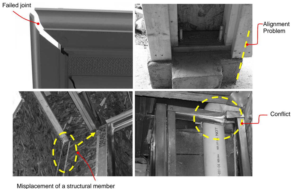
**Figure 5-11 : Typical Physical Interface Failures**
