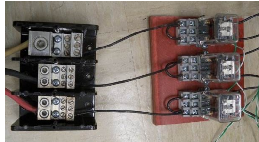
Fig. 4.71: Three-phase relay used as the PCC switch
