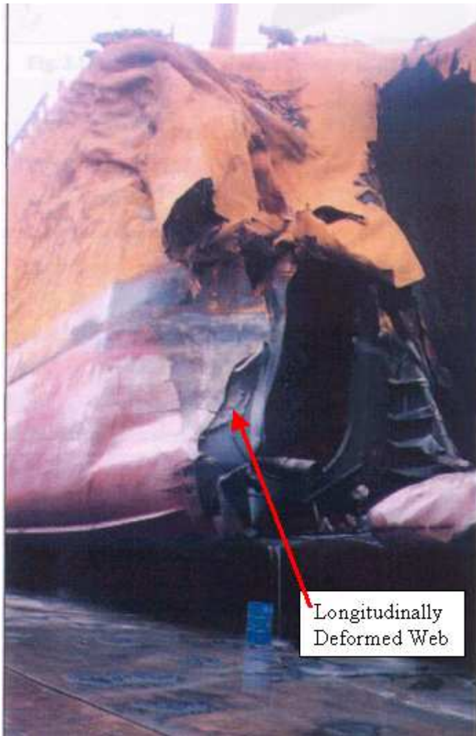
Figure 5-26 Actual Longitudinally Deformed Web [89]
