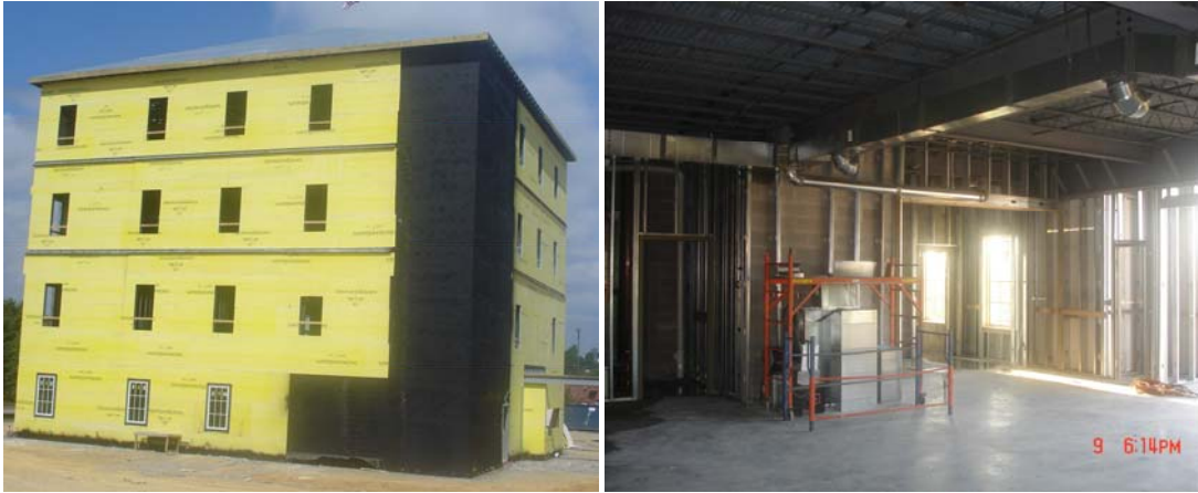
Figure 2.6: First Bank and Trust Building
