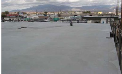
Figure 2.4: Long Span Composite Slab Mockup
