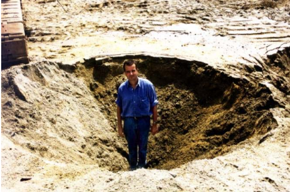
Figure 8-11. Conical surface depression created by vibrocompacting without backfill. (Photo courtesy of W.S. Degen, Vibro Systems, Inc.).
