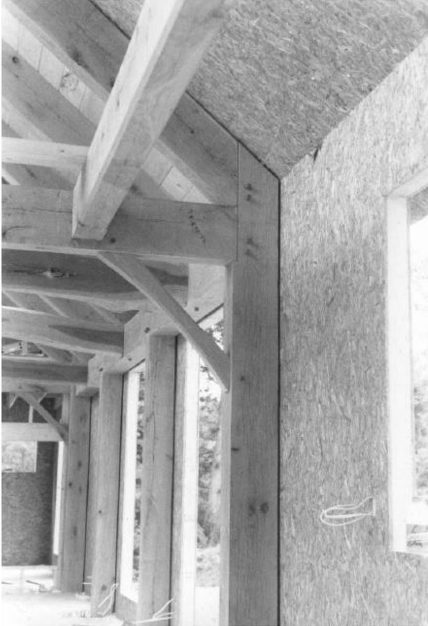
**Figure 1.2. Contemporary timber frame interior with SIP walls and roof is shown during construction. One inch (25 mm) oak pegs can be seen at the top of 8 in. (203 mm) by 10 in. (254 mm) post. Spacers between timbers and SIPs provide space for installation of drywall on walls and ceiling.**
