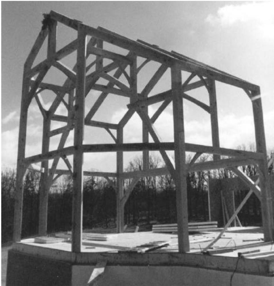
**Figure 1.1. Timber framing shown for a great room near Blacksburg, VA. The nominal timber sizes typically range from 6 in. (154 mm) by 6 in. (154 mm) to 12 in. (305 mm) by 12 in. (305 mm) and common species include Southern Pine, Douglas Fir and Mixed Oak.**
