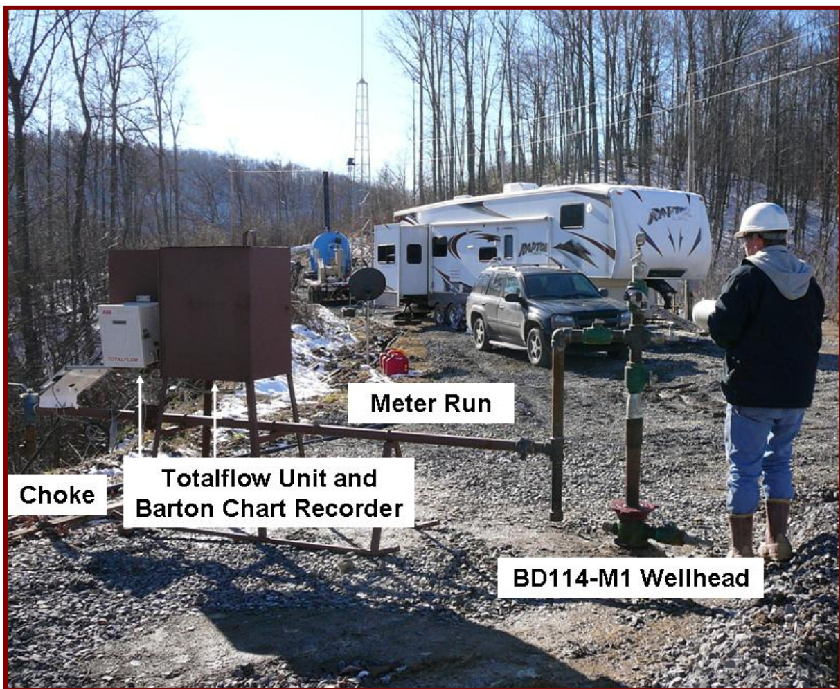
Figure 4.7 BD114-M1 Instrumentation
