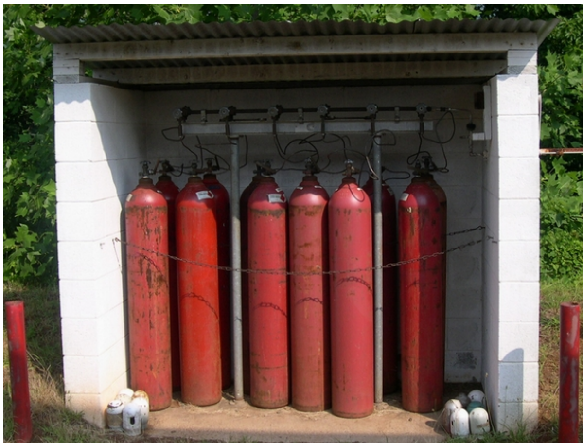
Figure 2.2. UVa fuel farm. Visible is the manifold which can hold up to twelve cylinders of fuel.
