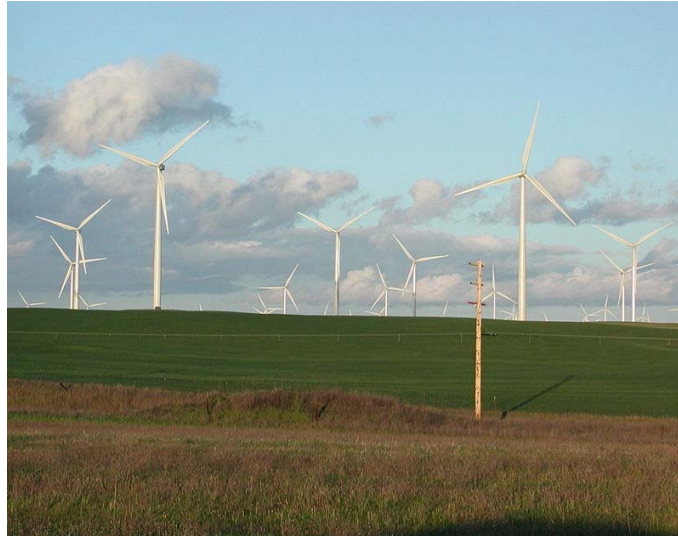
Figure 1.5 a) Onshore wind farm
