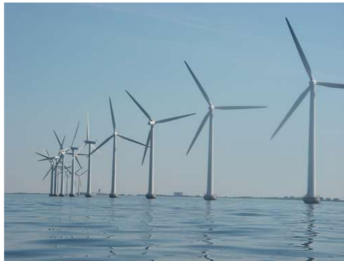
Figure 1.5 b) Offshore wind farm
