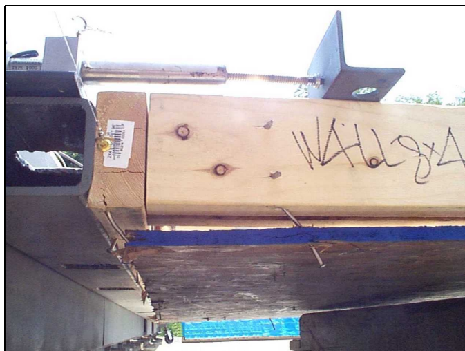
Figure 5. 19. Nails pull out of wood near the corner.
