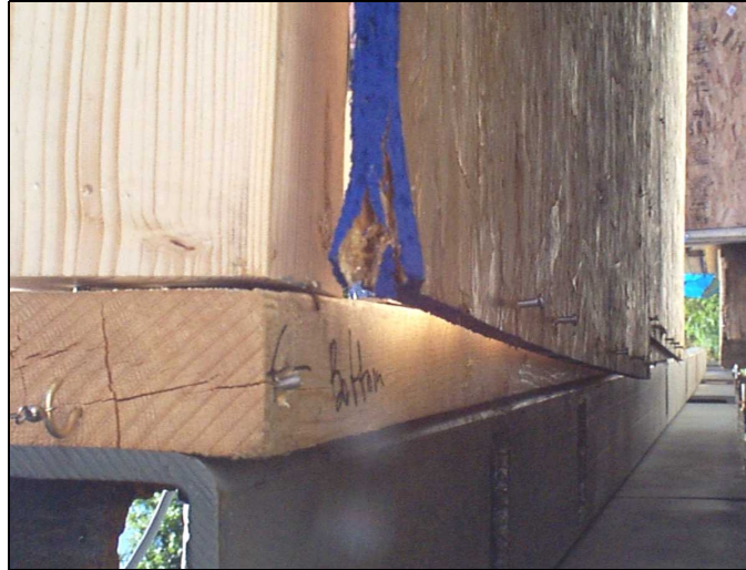
Figure 5. 17. Nail fatigue along the bottom plate in FAc wall.
