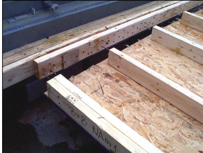
Figure 5. 46. Wall NAc1 after the test.
