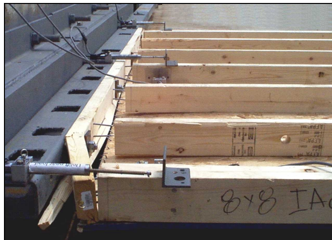
Figure 5. 37. Failure of 08Iac2re wall.
