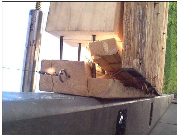
Figure 5. 27. Failure mode of 02IAM1re wall.
