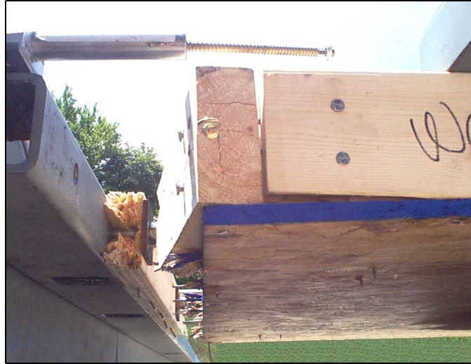
Figure 5.33. Failure of 04IAc1 wall.
