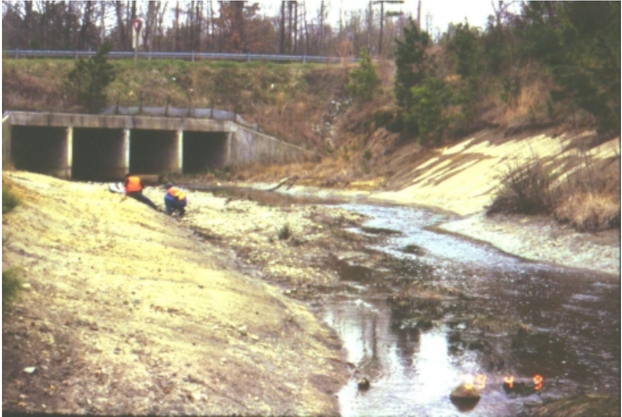
Figure 3.4. Proctor's Creek was redirected due to road construction near the intersection of Rts-288 and 156 in Chesterfield County. The creek was routed into an excavated channel through Lower Tertiary deposits. Extremely acid soil conditions ( \text{pH} < 2.5 ), which developed upon oxidation of the sediments, have inhibited vegetation along the stream bank.
