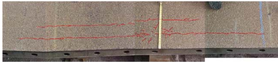
(a) South edge cracking of the surface overlay
