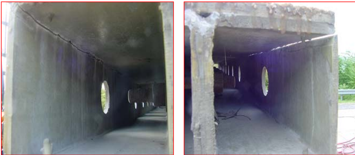
Figure 5.26 Damage of the internal tubes at the free edges
