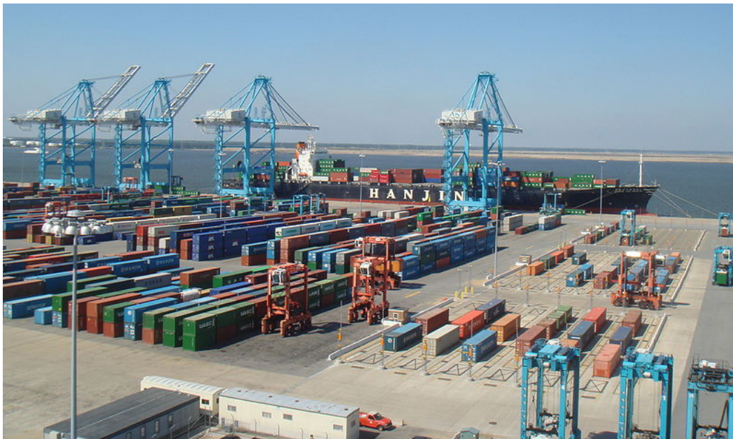
Figure 5-14. Example of a Container Terminal [55] (Missy Schmidt. Wikipedia. [Online]. http://en.wikipedia.org/wiki/File:Norfolk_International_Terminal.jpg , Used under fair use guidelines, 2011.)
