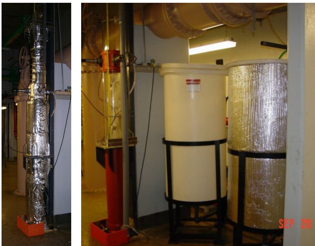
Figure 3.1 Pilot reactor with a feed tank and a spare holding tank before insulation (right) and after insulation (left). The un-insulated tank served as a holding tank for centrate.
