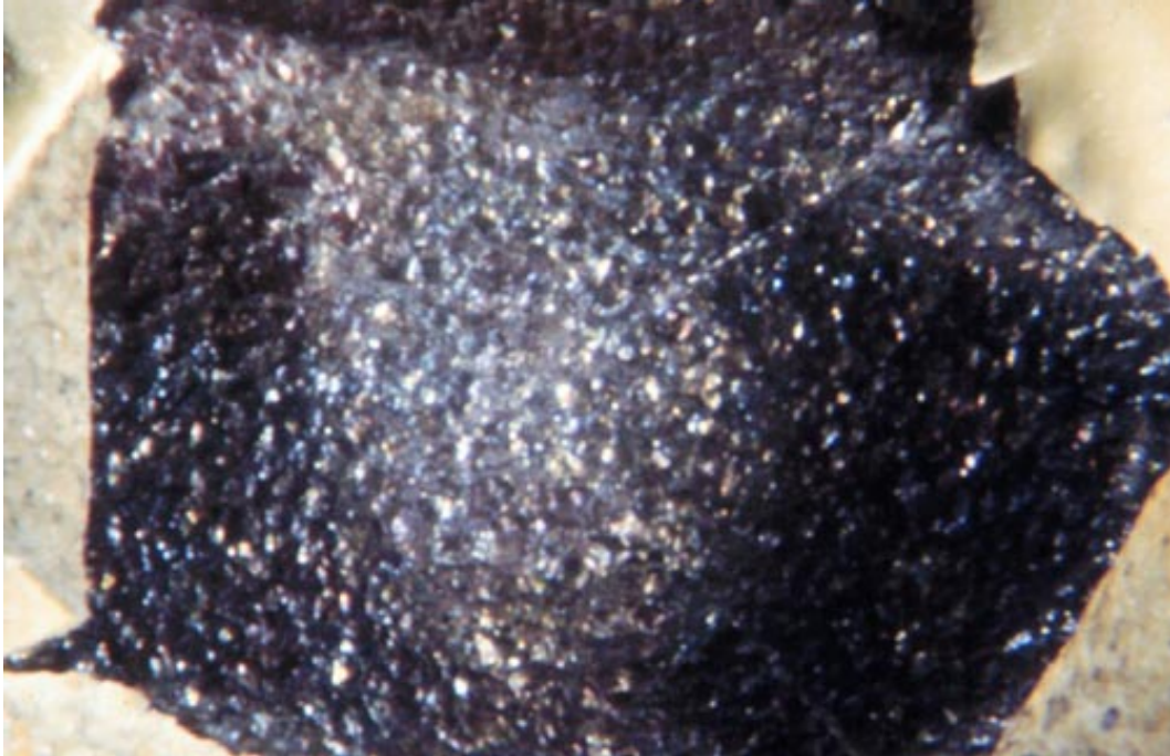
Figure 44. Black, Shining Steel Surface Underneath Coating.
