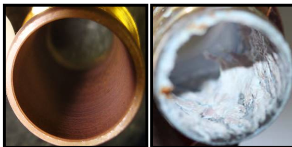
Figure 5.1: Dezincified interior (left) and meringue build-up (right) within brass plumbing components.
