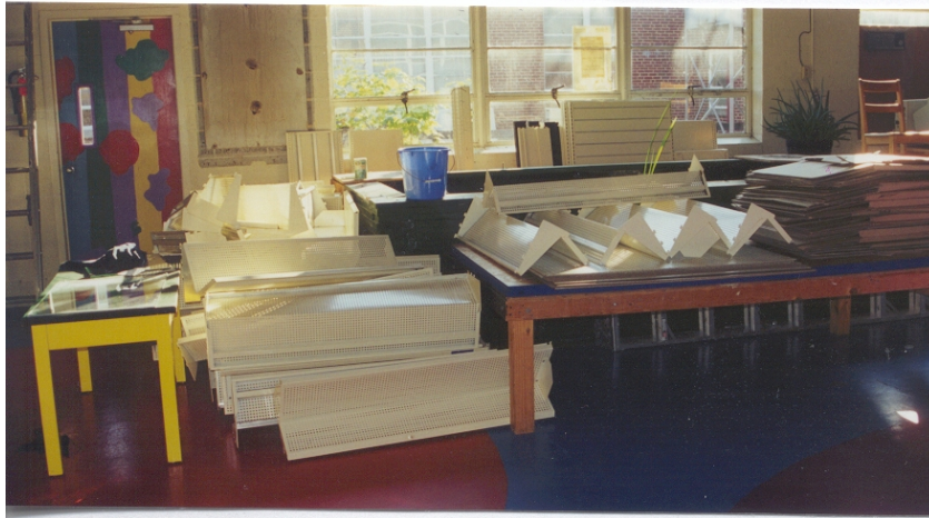
Figures 3 and 4. Studio renovation
