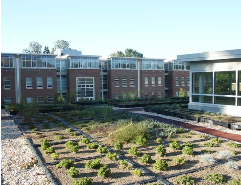
GreenTech modular green roof atop the Tucker-Brand Middle School Art Building
