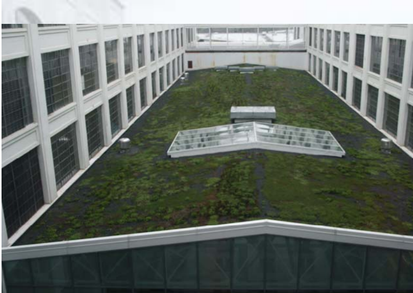
20,000 SF green roof on the main building
