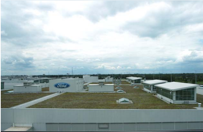
The green roof atop the new truck plant retains approximately 50% of incident rainfall.
