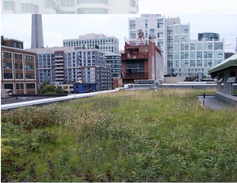
The green roof reduces temperatures at the roof surface.
