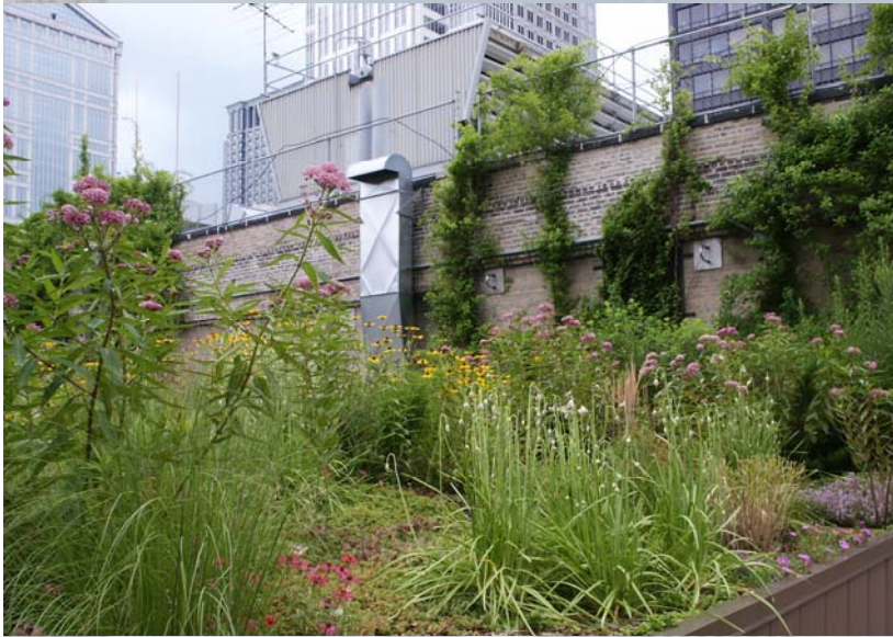
The green roof trims the load off traditional HVAC systems.
