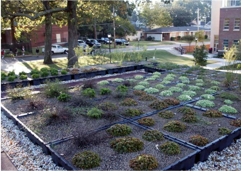
Modules are clearly visible on roof surface
