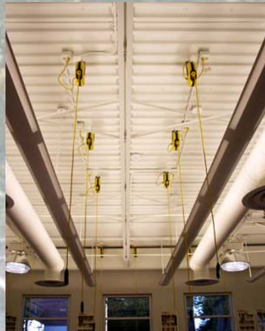
Underside of roof deck in Art Building
