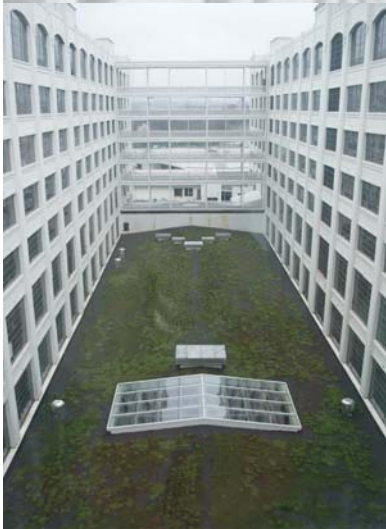
Adaptive re-use of the 1920s structure
