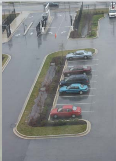
Bioretention after a day of steady rainfall
