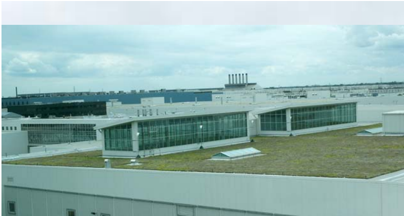
Roof monitors bring natural light to factory space.
