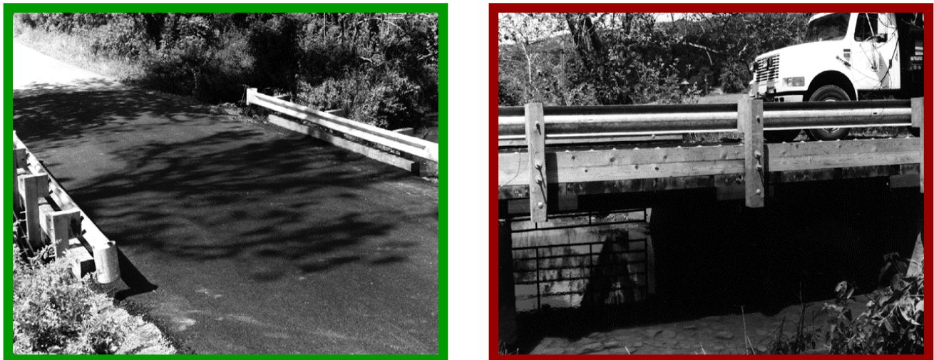
Figure 2- 22. Tom’s Creek Bridge (front and side view)
