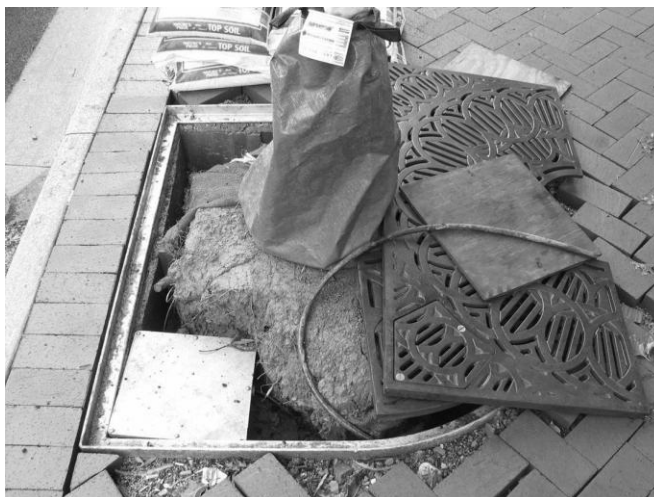
Figure 2.1 A bad example of a street tree planting; downtown Blacksburg, VA. The root ball has been trimmed to accommodate for a utility box, the planting pit is very small thus providing only little soil for the tree and the planting pit is aligned with concrete to contain the roots. The growing condition for this tree is poor jeopardizing the survival potential of the tree.
