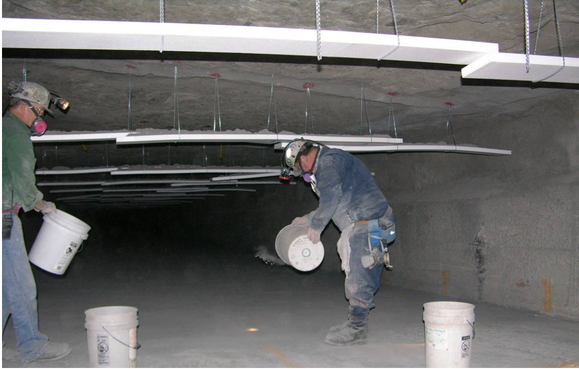
Figure 3.21 – Example of the coal and rock dust being suspended from the mine roof and placed on the mine floor.*
