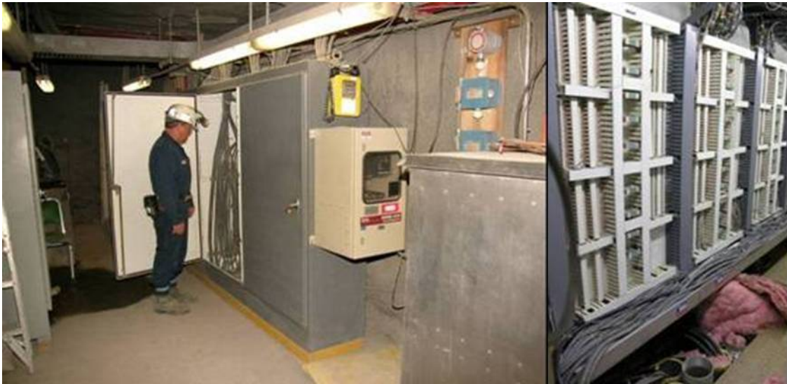
Figure 3.6 – View of the panels inside (left) and outside (right) of the mine which contain corresponding wire terminals.
