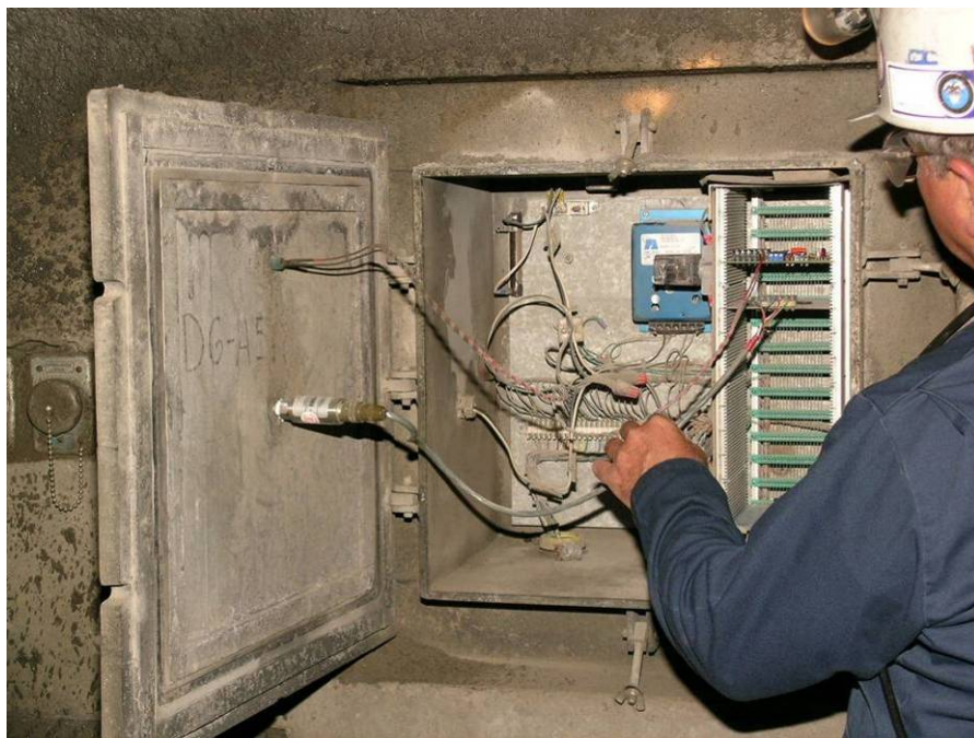
Figure 3.7 – Data gathering station located in one of the mine drifts.*
