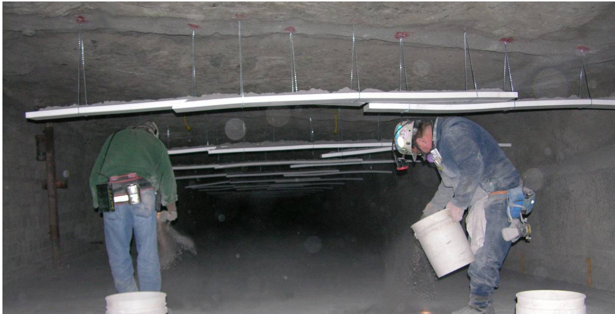
Figure F.12 – Photograph of the mine shelves and chains used in the series of mine shots with different rock and coal dust concentrations.
