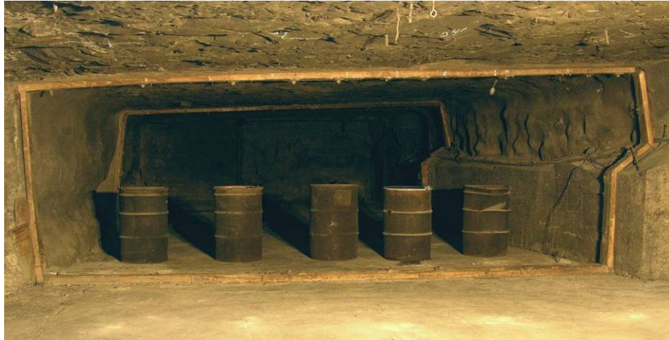
Figure 3.19 – Ignition chamber located at the end of C-Drift.*
