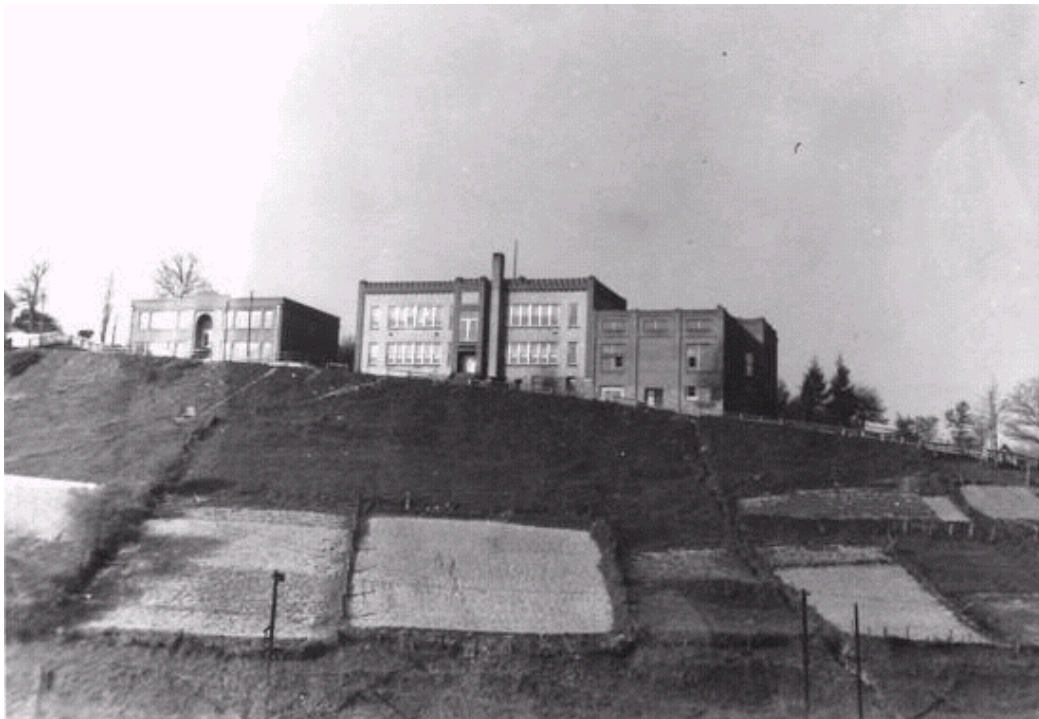
The expansion of Pocahontas High School during the late 1920s led to the addition of Pocahontas Elementary School (left) and the first gymnasium/auditorium in Tazewell County (right). (Photo courtesy of the Library of Virginia)
