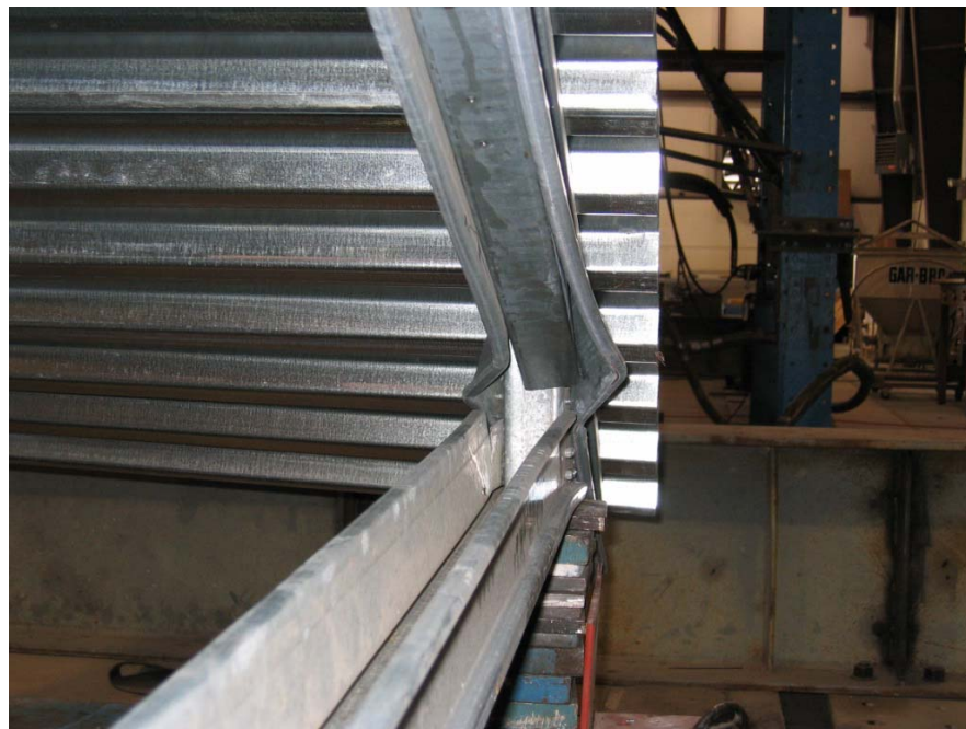
Figure 5.10 T1C Test 2 Local Buckling Failure
