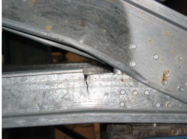
Figure 5.11 T1C Test 2 Fracture after Local Buckling Failure
