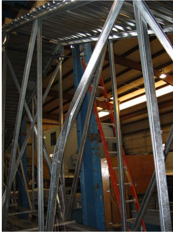
Figure 5.4 T1A Test 1 (First Run) Out-Of-Plane Buckling
