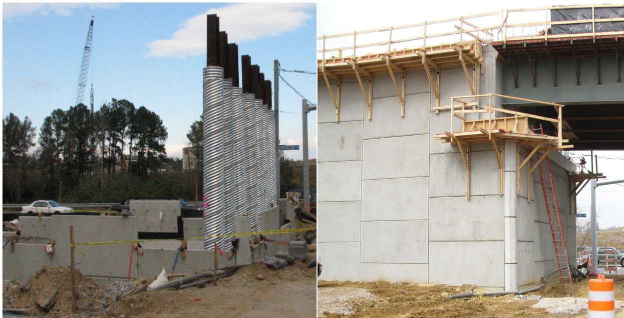
Figure 7.1 – Telegraph Road Bridge in Alexandria, VA. Left: Abutment B672 under construction, showing concrete panels, foundation piles, and corrugated steel sleeves. Right: Abutment B672 almost completed, showing concrete panels, girders and abutment.
