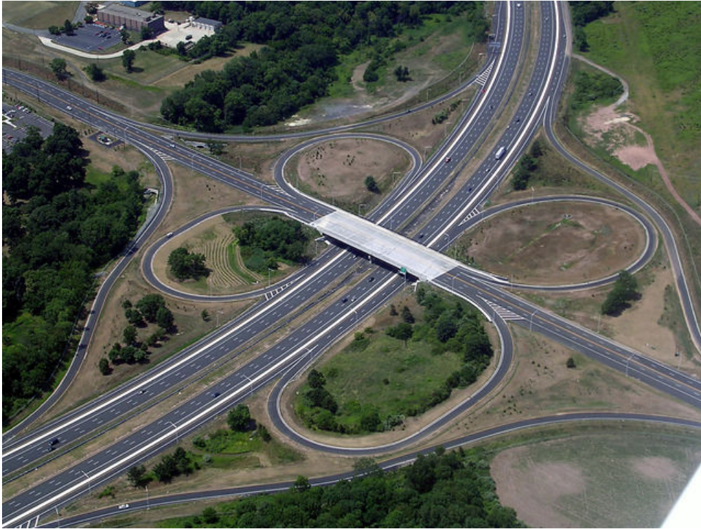
Figure 6.1 – Scotch Road integral abutment bridge
