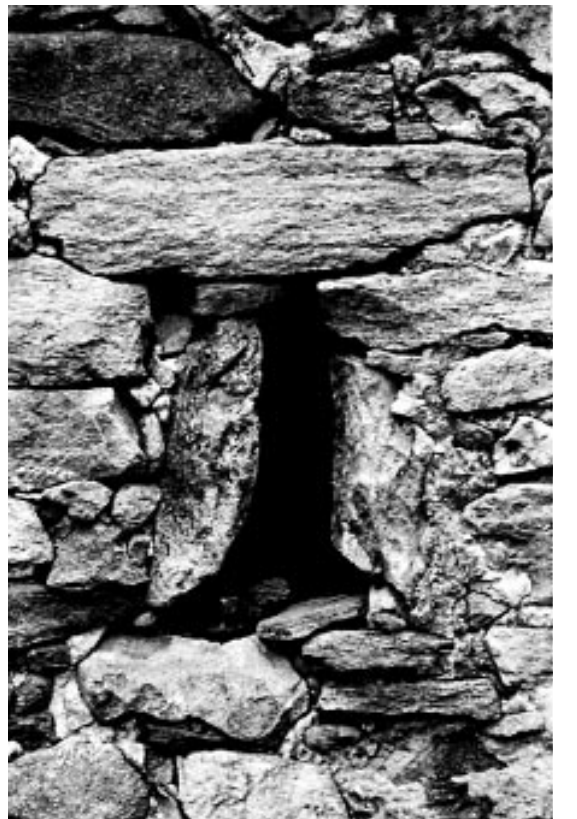
wall opening, close view (2.52)
