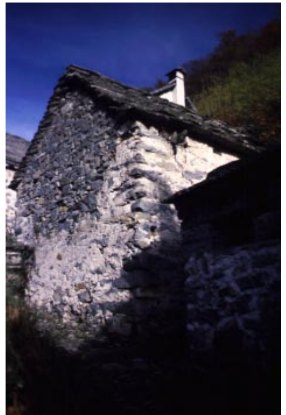
massive dwelling in hill side (2.35)
