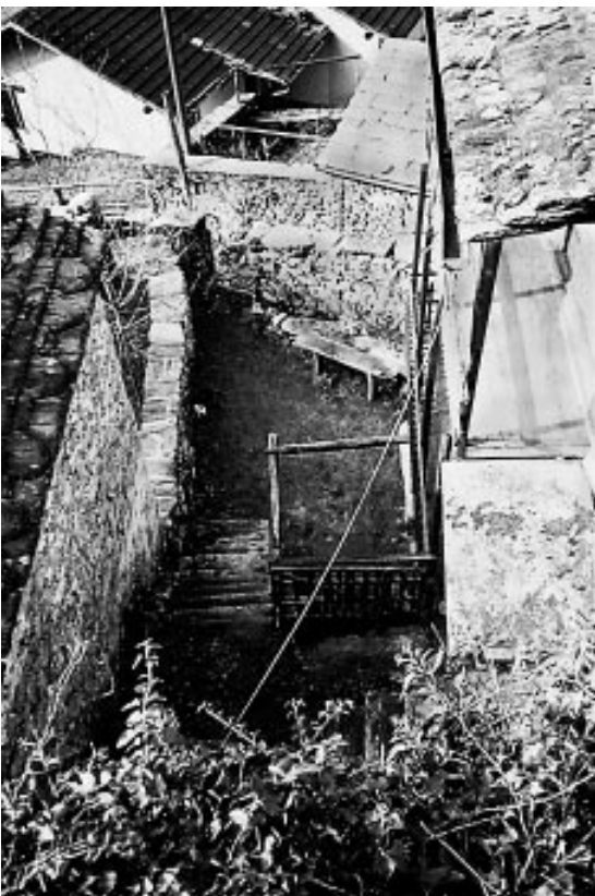
view down into courtyard (2.53)
