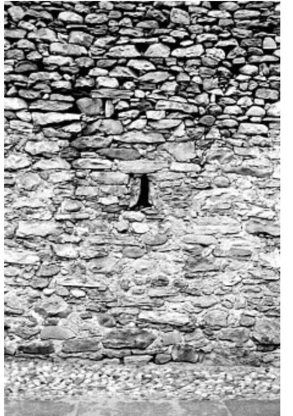
wall opening, middle view (2.48)
