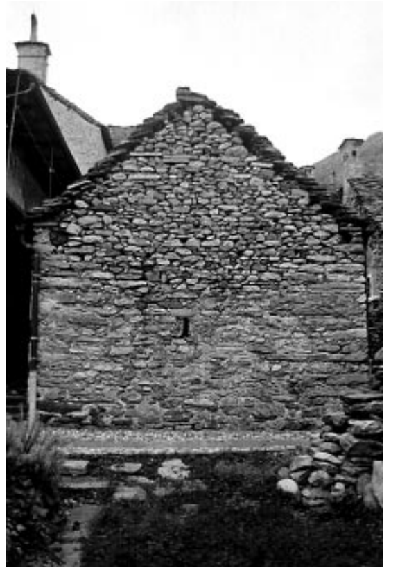
wall with single opening, distant view (2.44)
